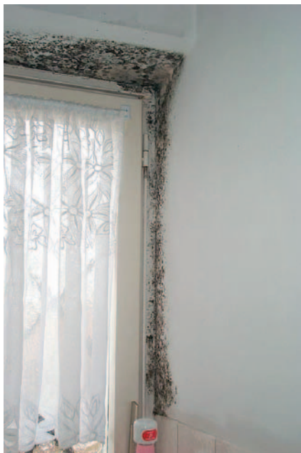
Mould infestation after water damage. Mould fungi are not only an aesthetic problem but also a health risk!
