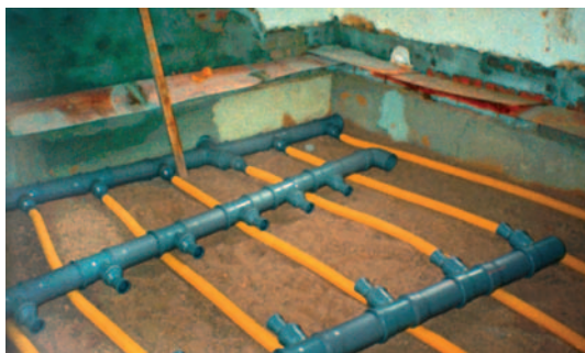
Installation of a drainage system beneath the foundations (here during the construction of the building) with the aim of extracting soil air containing radon and venting it out of the building.
